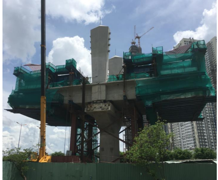
One of HCMC's many partially completed metro sites (Source: Internal)
