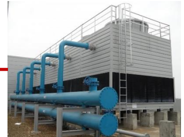
Cooling Tower Variable speed
